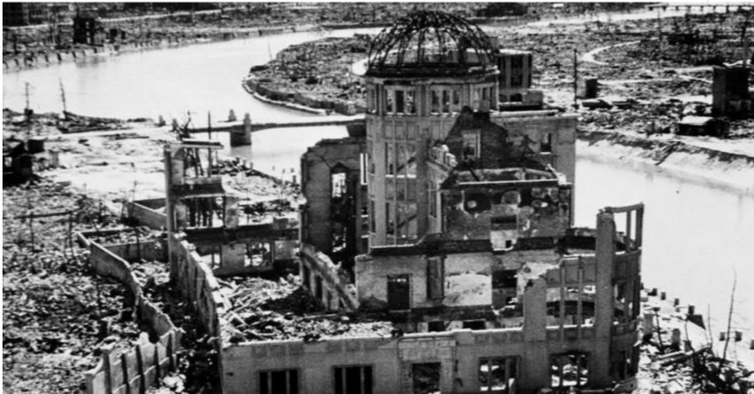
The remains of the Prefectural Industry Promotion Building, after the US dropping of the atomic bomb in Hiroshima, Japan. This site was later preserved as a monument.
