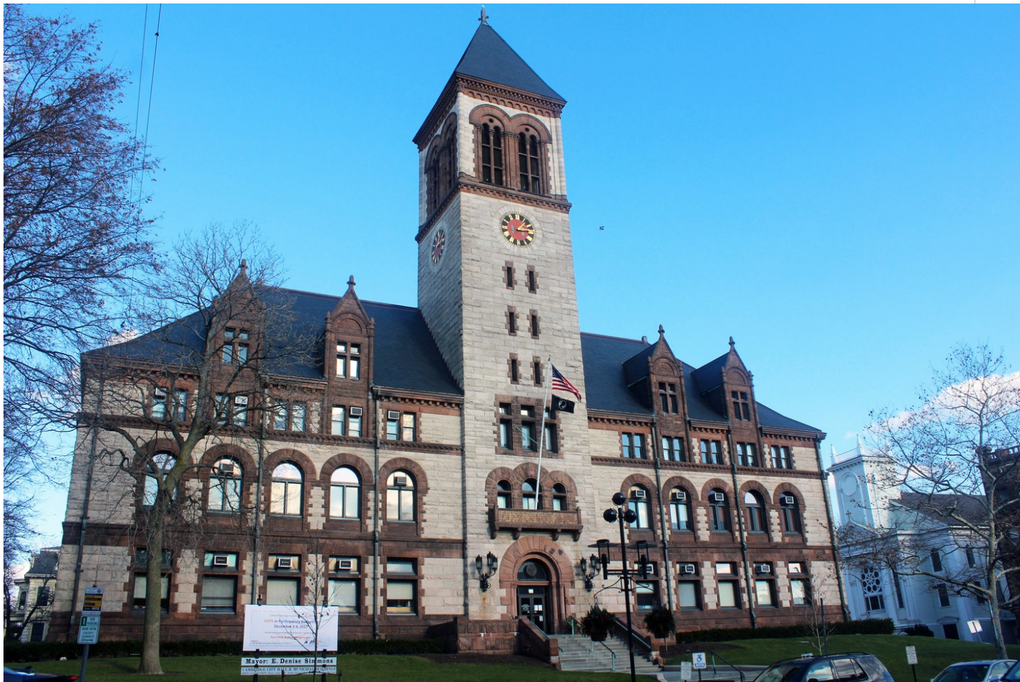
City Council Building, Cambridge, Massachusetts.
