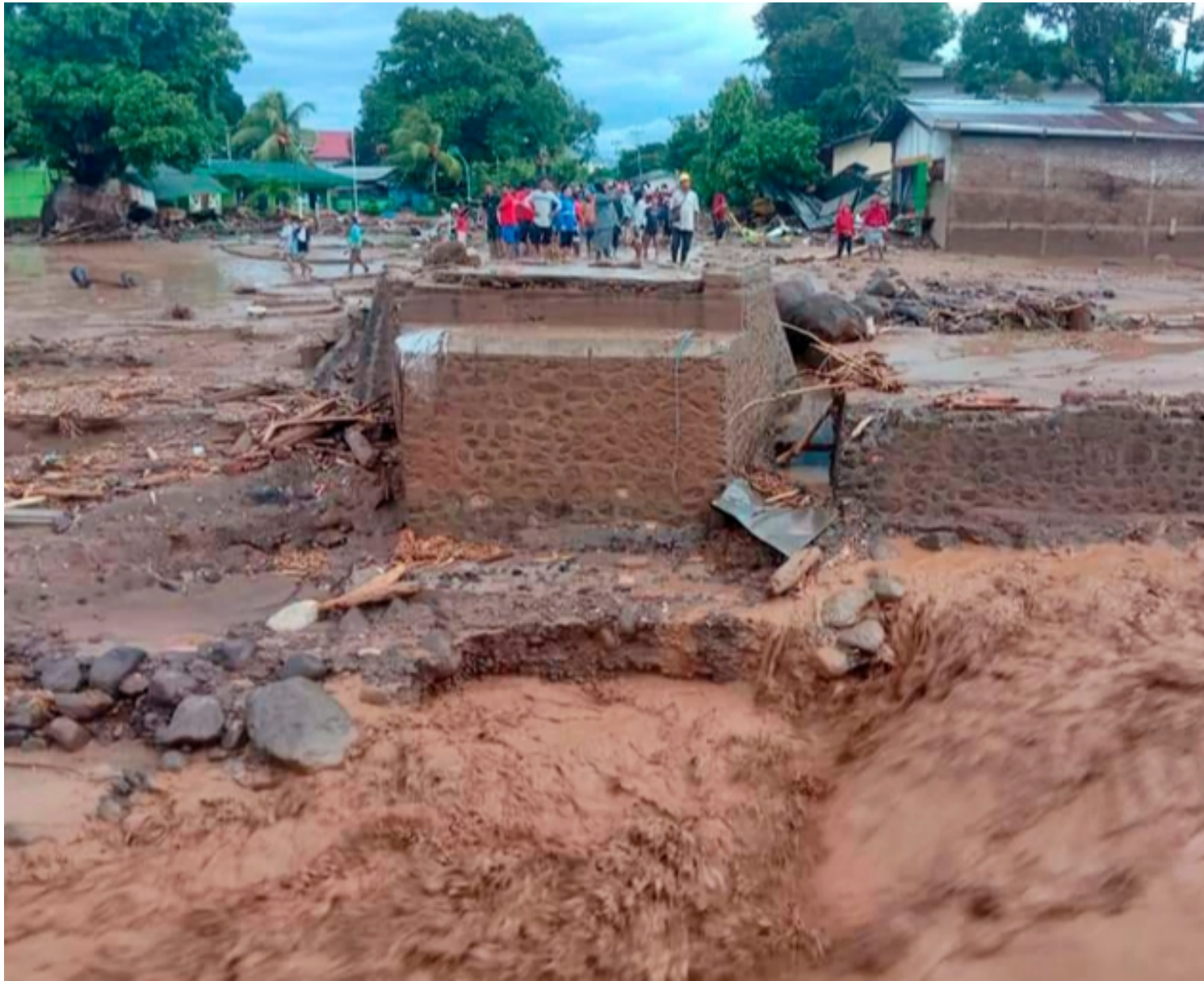
People inspect damaged buildings at a village hit by flash flood in East Flores, Indonesia [Photo: Ola Adonara/AP]
