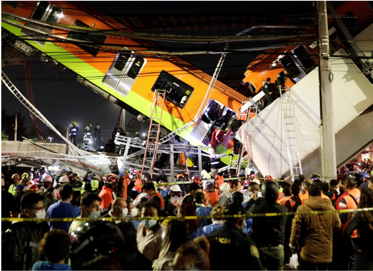
Rescuers work at a site where an overpass for a metro partially collapsed with train cars on it at Olivos station in Mexico City late Monday night. (Photo: Luis Cortes / Reuters)
