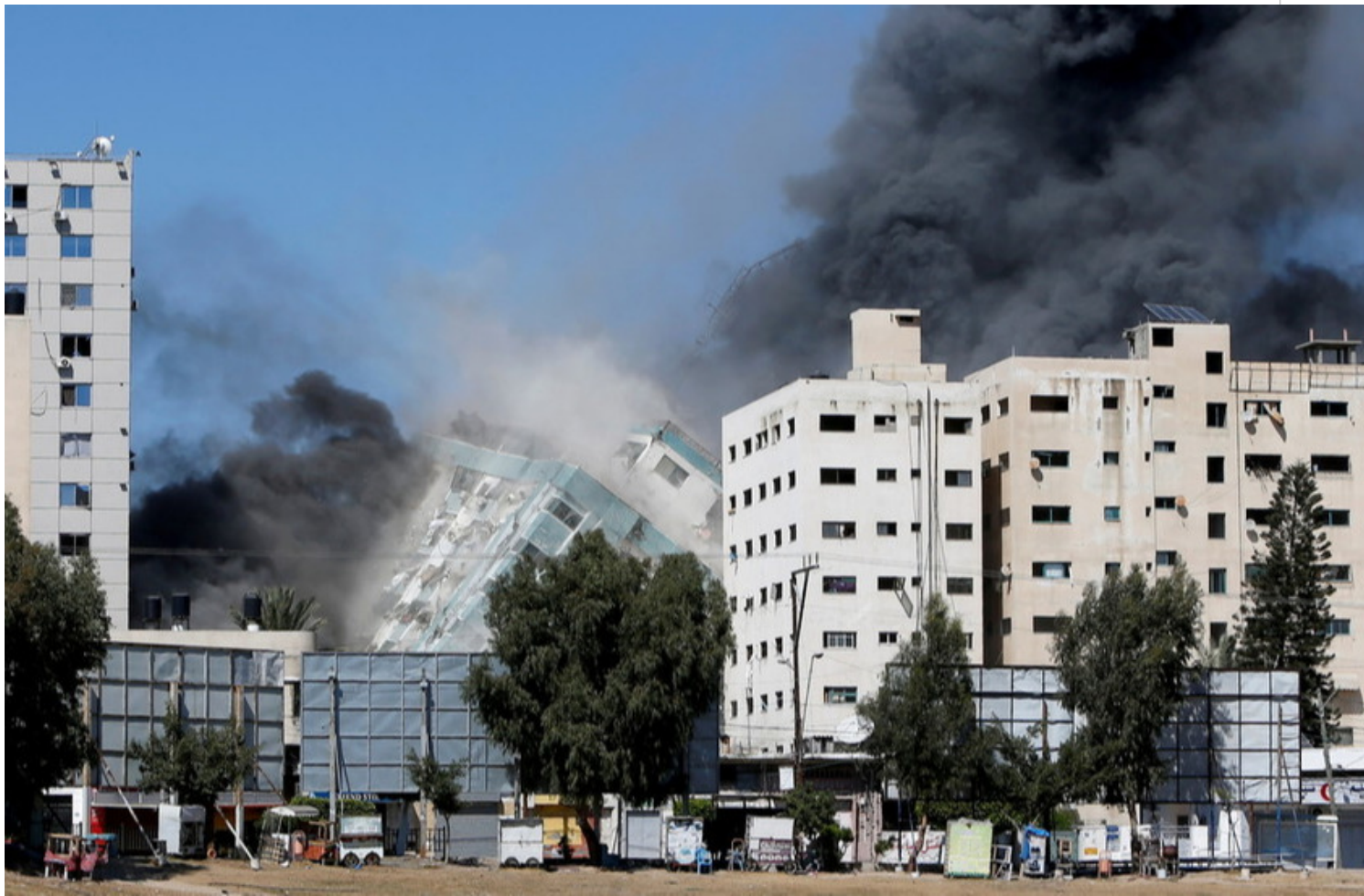
A tower housing AP, Al Jazeera offices collapses after Israeli missile strikes in Gaza City. (Photo: Reuters / Mohammed Salem)
