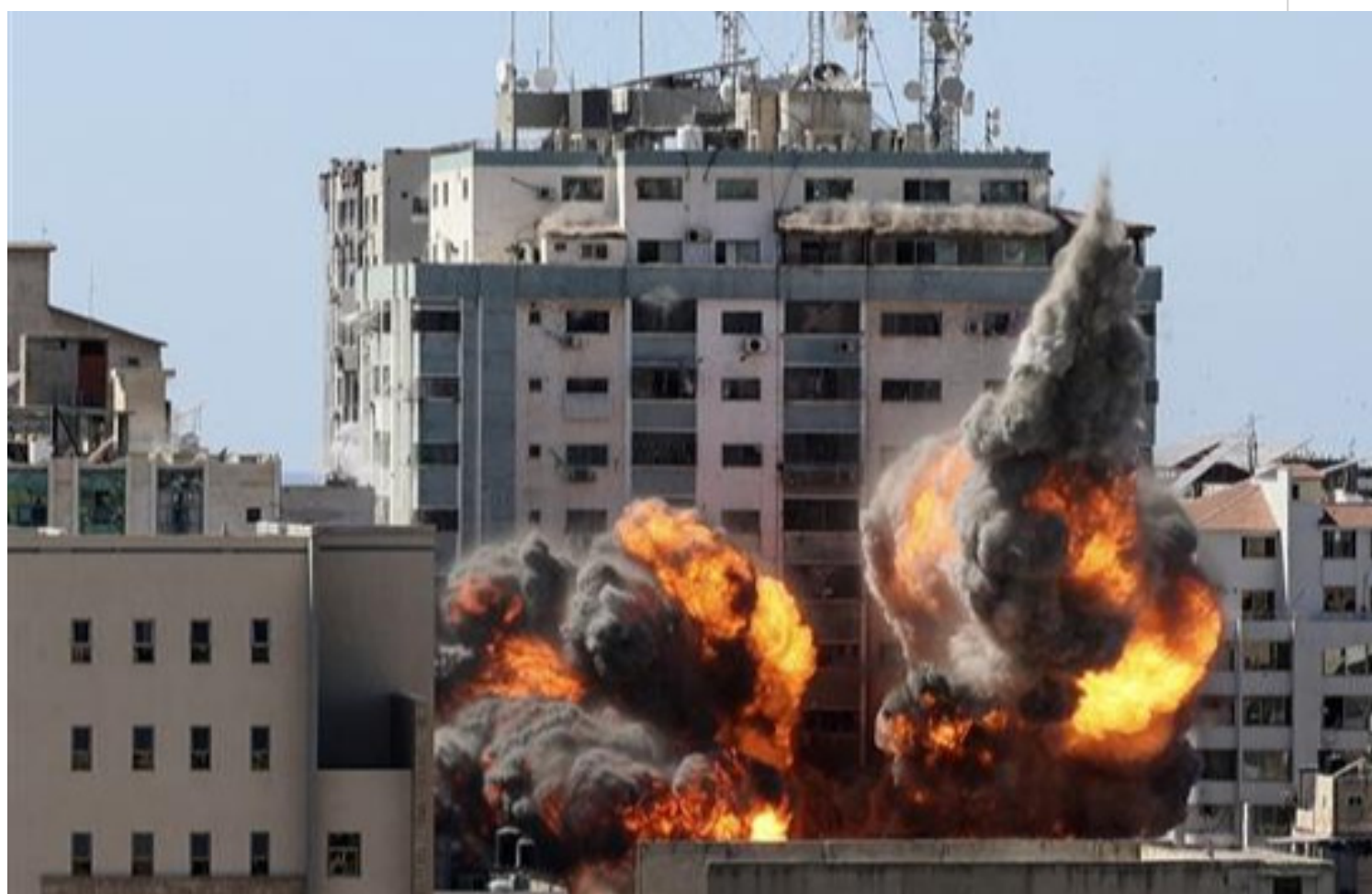
Fire and smoke rises from the al-Jalaa Tower as it is destroyed in an Israeli airstrike on Gaza City, on May 15, 2021. (Photo by AFP)
