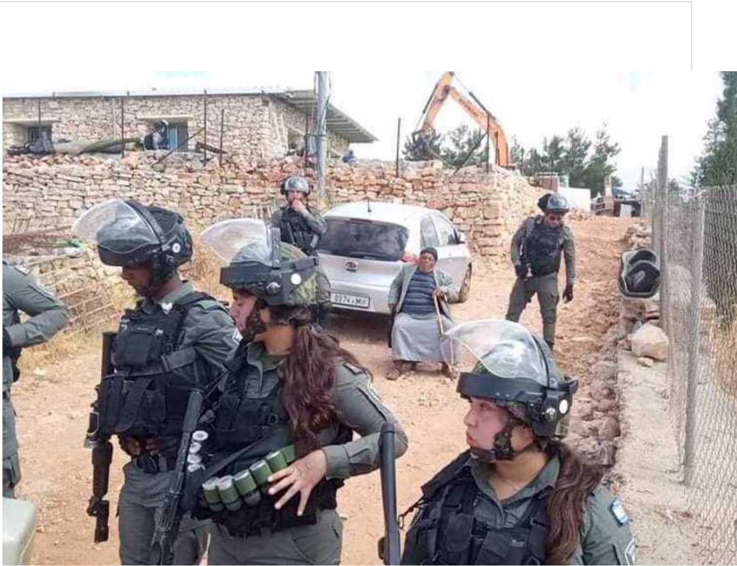
Israeli forces surround a house and a tract of agricultural land before demolition in the occupied West Bank on June 17, 2021. (A photo by Palestinian WAFA news agency)
