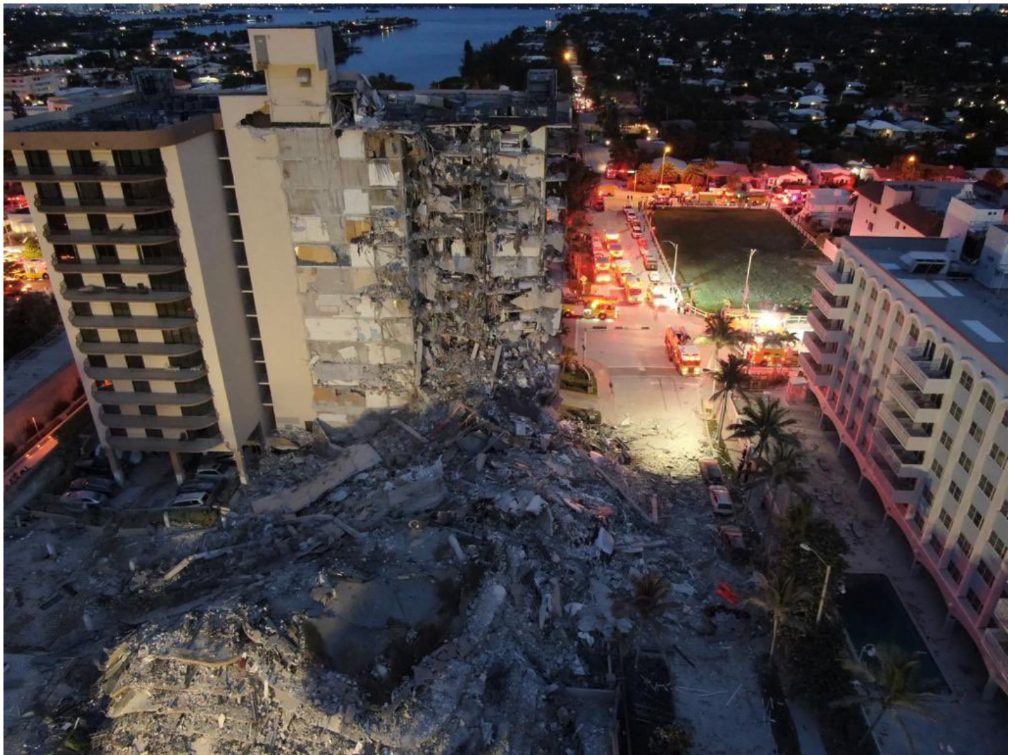
Havana, July 1 (RHC)—Cuba conveyed its condolences to the relatives of the victims of the partially collapsed building in Surferside, Florida.
