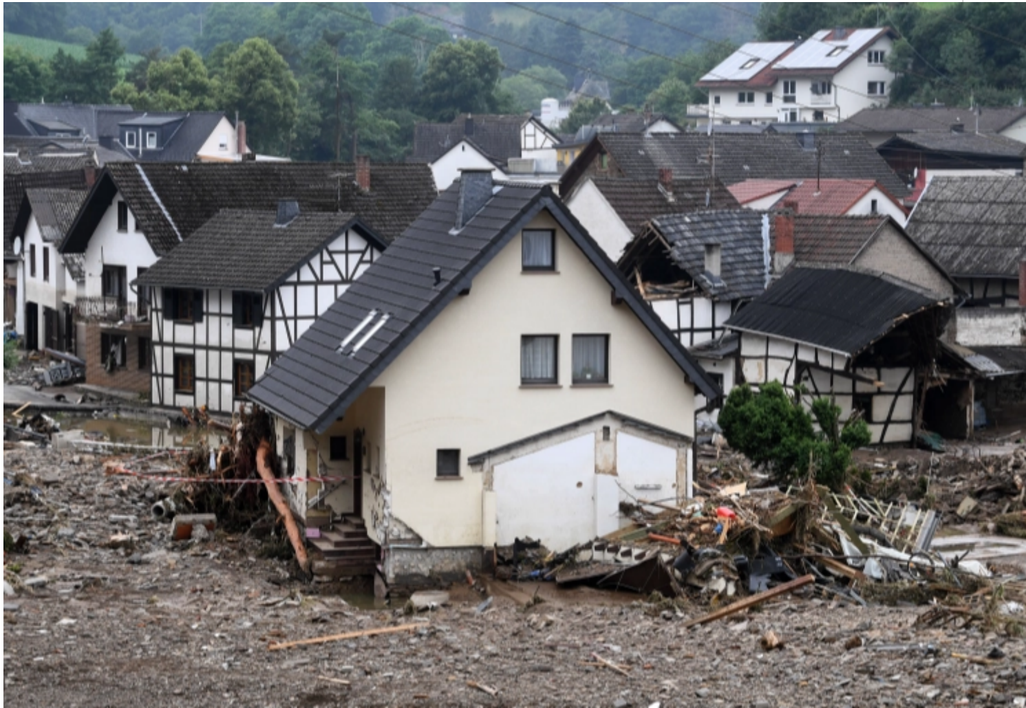
Destroyed houses are seen after floods caused major damage in Schuld near Bad Neuenahr-Ahrweiler, western Germany [Photo> Christof Stache/AFP]
