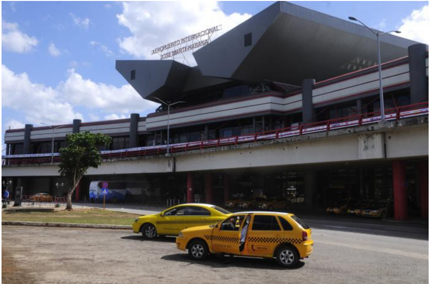
Havana's Jose Marti International Airport
