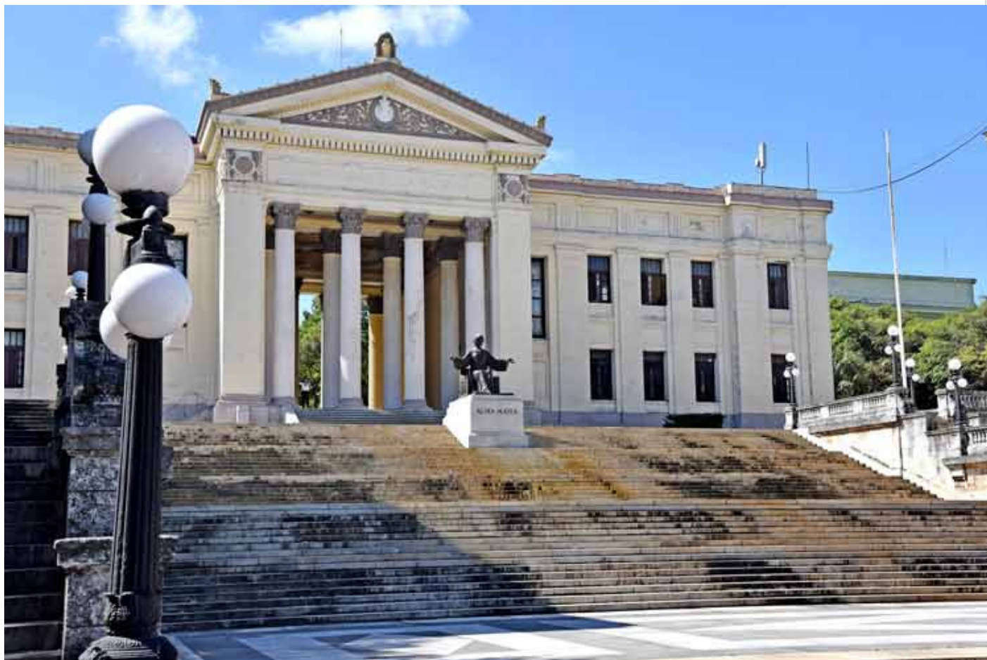
Havana's University main entrance.
