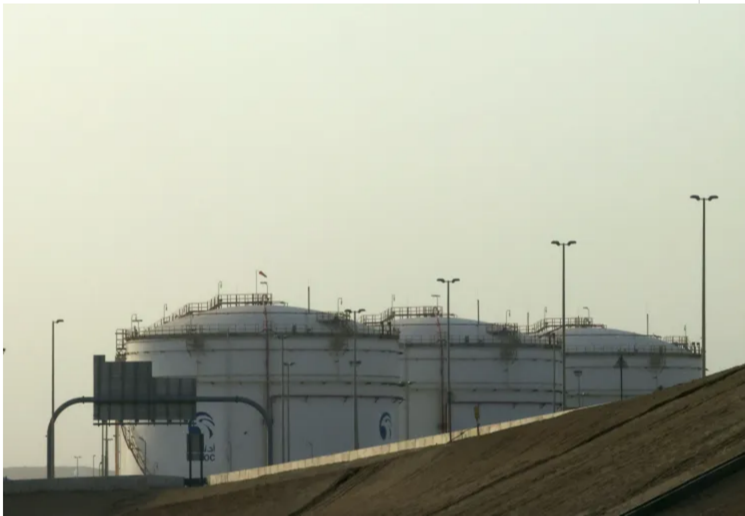
A picture shows a storage facility of oil giant ADNOC in the Msaffah industrial district in the Emirati capital Abu Dhabi
