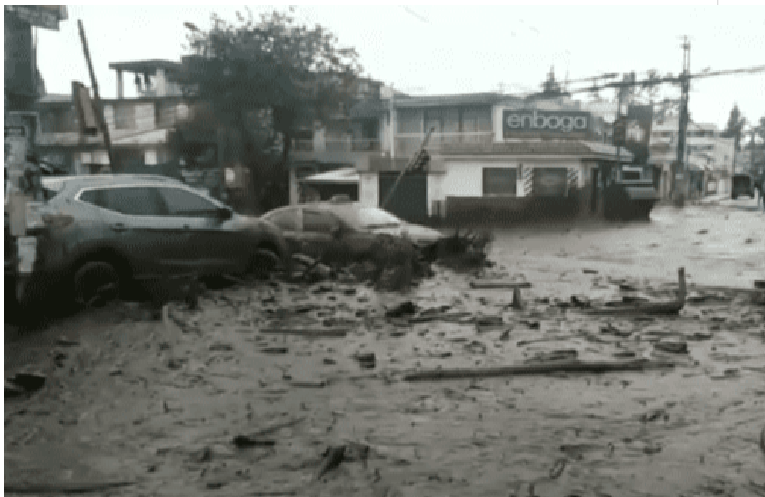
The flooding caused by heavy rains in La Gasca caused damage to the electric power system and infrastructure. | Photo: La Hora
