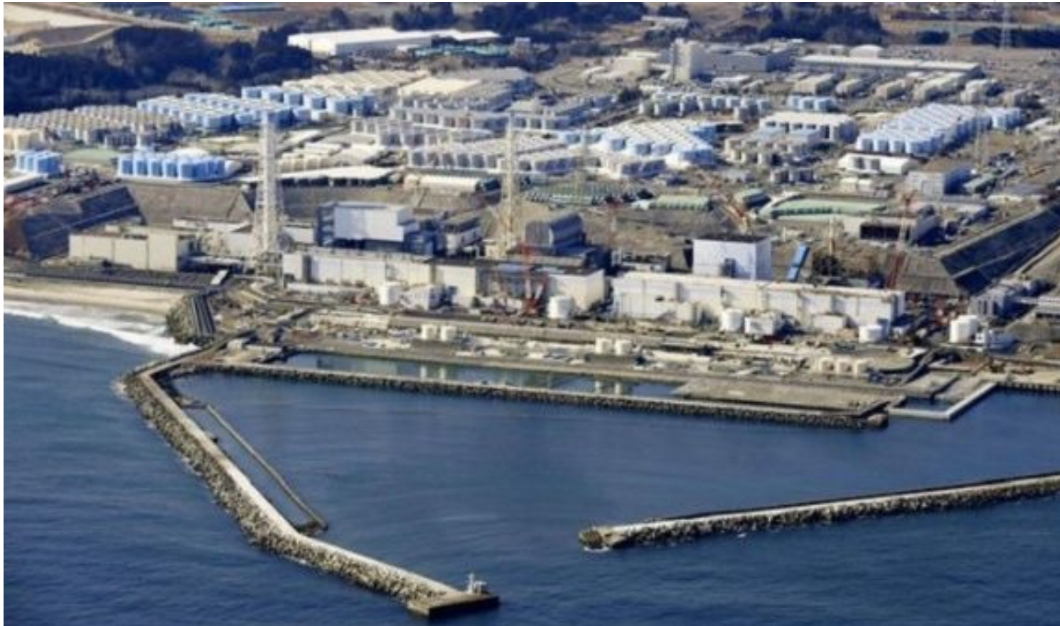
Fukushima Daiichi Nuclear Power Plant, Japan, 2022. | Photo: Twitter/ @PDChina
