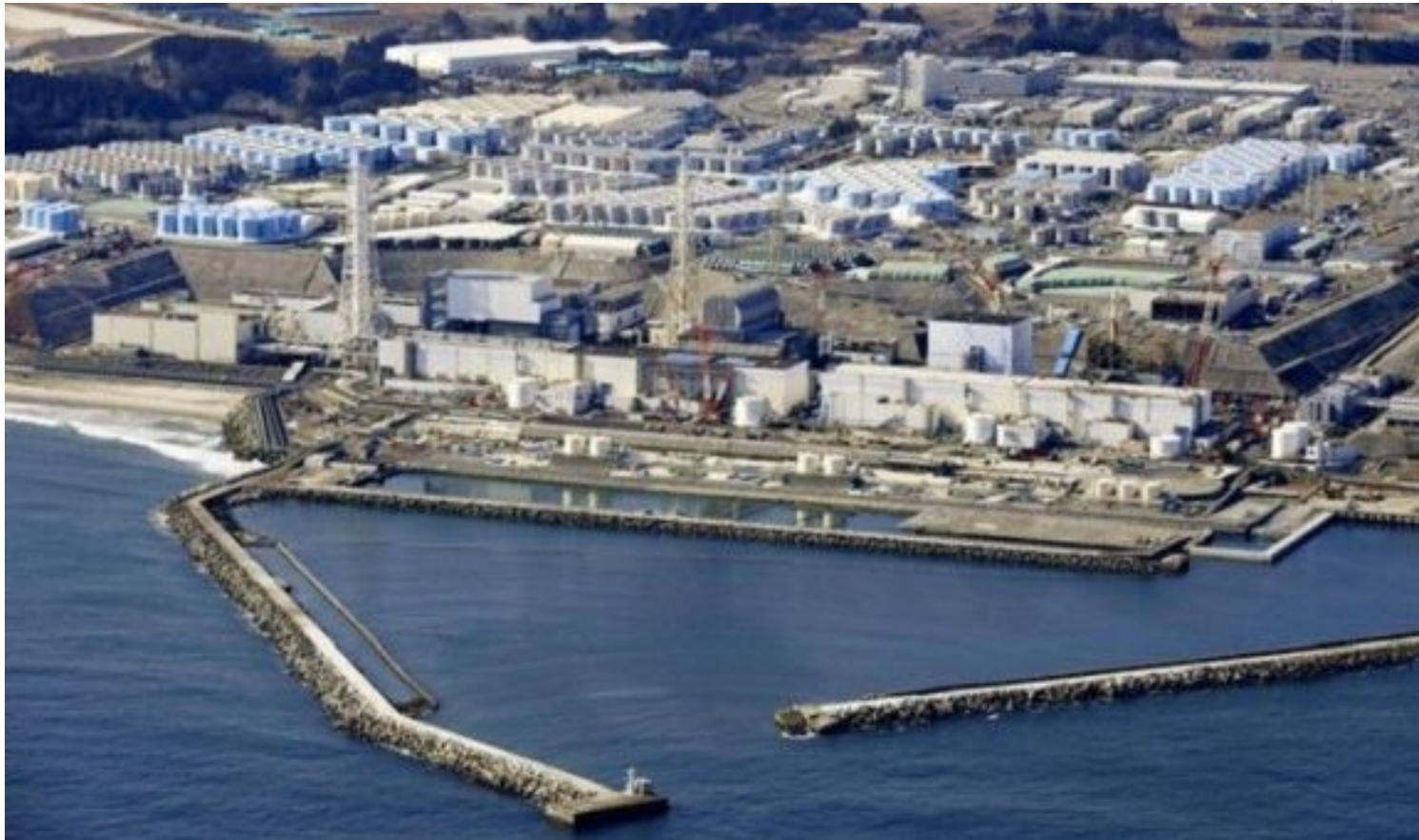
Fukushima Daiichi Nuclear Power Plant, Japan, 2022. | Photo: Twitter/ @PDChina
