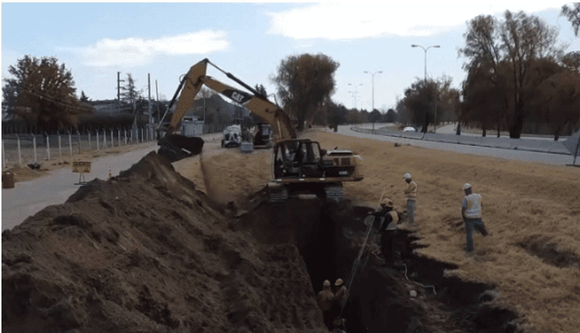
Workers at a Great Argentina's project site. | Photo: Twitter/ @gkatopodis
