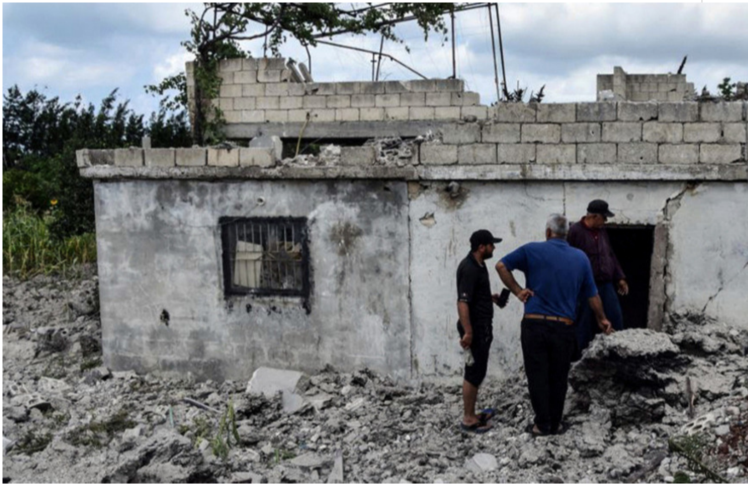
This handout picture released by the official Syrian Arab News Agency on July 2, 2022, shows men assessing the damage caused to a building by an Israeli airstrike in the western Syrian coastal city of Tartus. (Via AFP)
