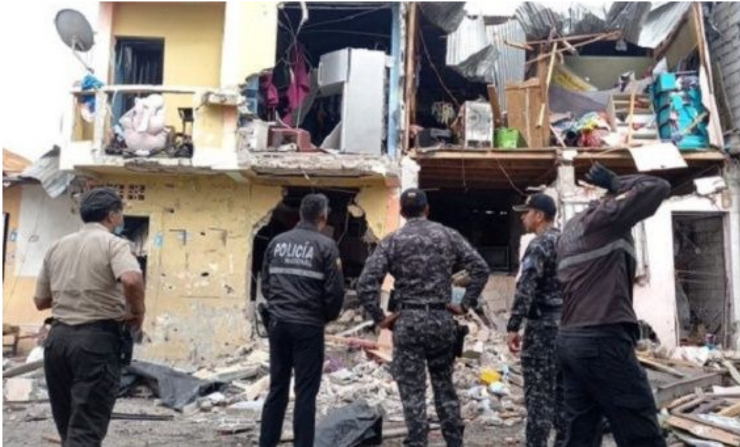
Houses destroyed by the explosion, Guayaquil, Ecuador, Aug. 15, 2022. | Photo: Twitter/ @turkiyenews
