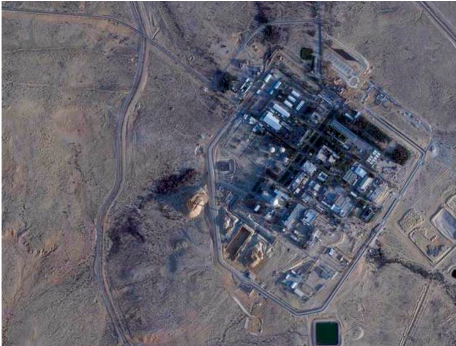
This satellite photo, released earlier this year, shows construction near the Shimon Peres Negev nuclear center, not far from the city of Dimona, in Israeli-occupied Palestine. (Via AP)
