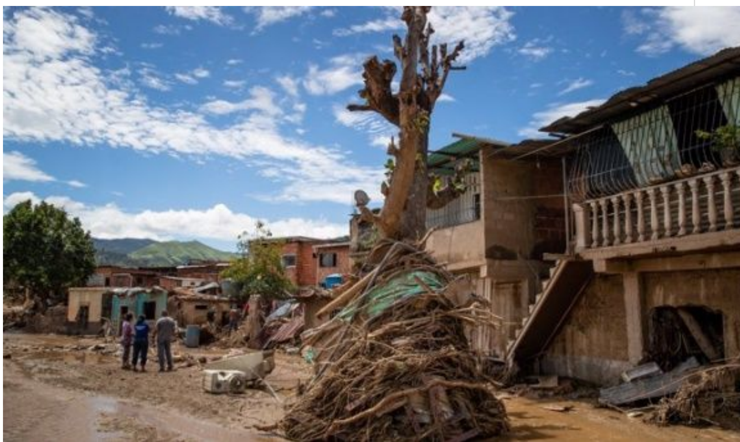
View of damage caused by the overflow of the Los Patos stream, in Las Tejerías, Aragua state | Photo: EFE/Miguel Gutierrez
