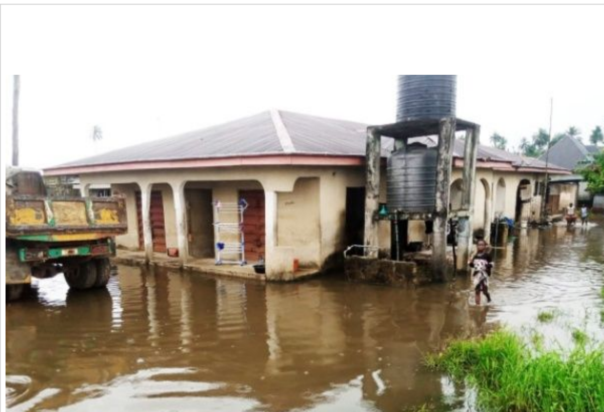
Photo taken on Oct. 9, 2022 shows flooded houses in the Ahoda West area of Rivers state, south Nigeria. | Photo: NAN via Xinhua
