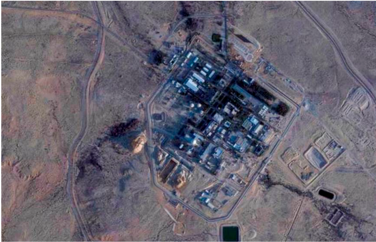
This satellite photo, released on February 22, 2021, shows construction near the Shimon Peres Negev nuclear center, not far from the city of Dimona, in Israeli-occupied Palestine. (By AP)
