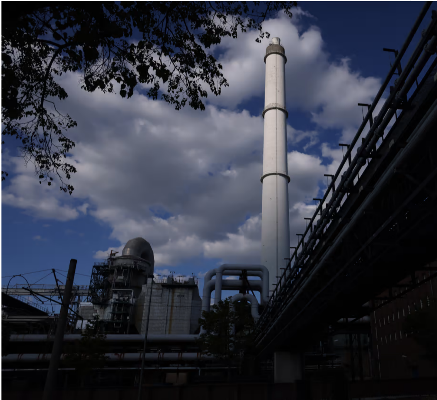
Klingenberg natural gas-powered thermal power station in Berlin, Germany (Via Getty Images)
