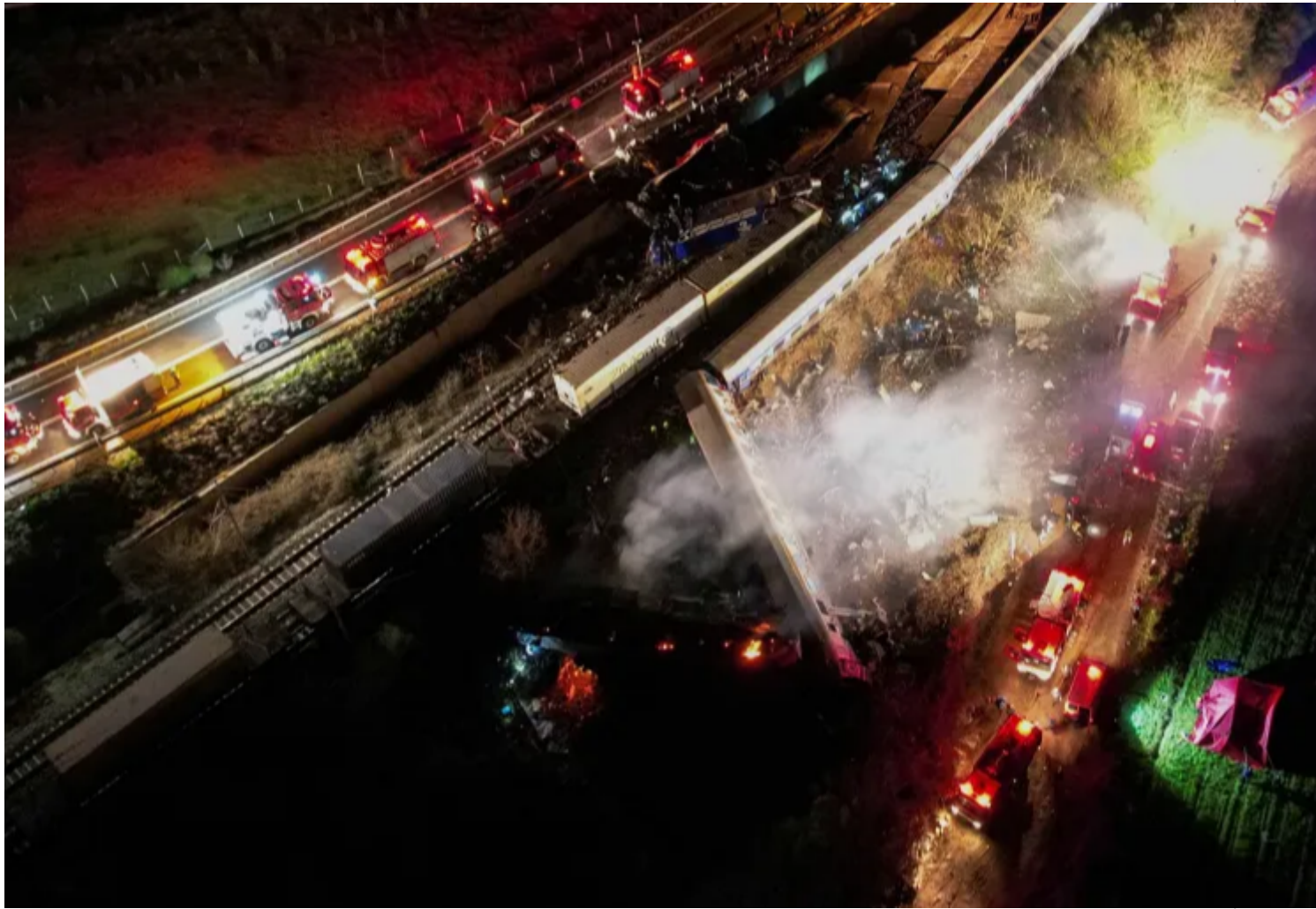
An aerial view of the site of the crash between a passenger train and cargo train in central Greece. The circumstances of the collision remained unclear [Giannis Floulis/Reuters]
