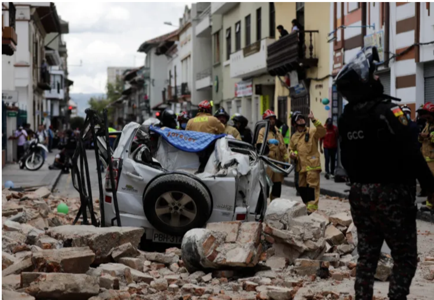
Magnitude 6.7 tremor shakes coastal Guayas region, damaging homes and buildings.
