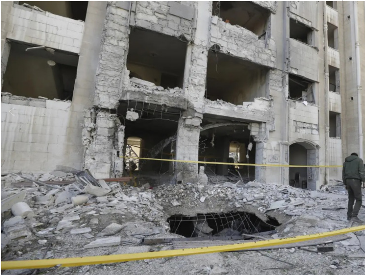
Syrian security officers inspect the damage in a residential neighborhood after an Israeli
