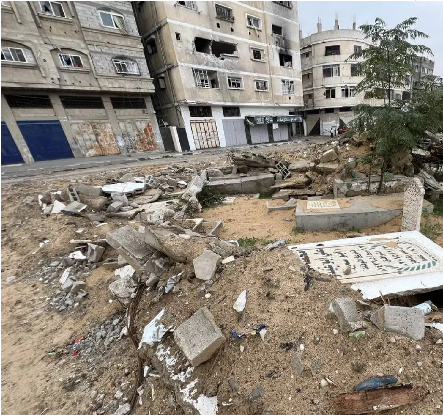
A view of destroyed the Fallujah cemetery, which it used as a headquarters by Israel military, and damaged buildings as Israeli attacks continue on Gaza Strip, on December 14, 2023. [Fadi Alwhidi – Anadolu Agency]
