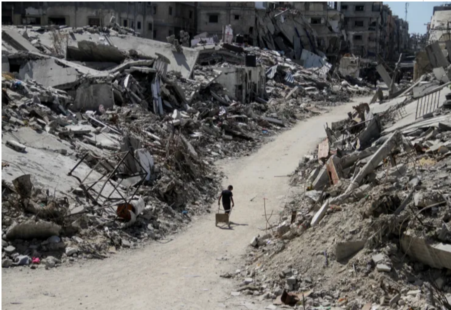
A Palestinian walks among the rubble of damaged buildings in Beit Lahiya, in the northern Gaza Strip, on Wednesday [Mahmoud Issa/Reuters]
