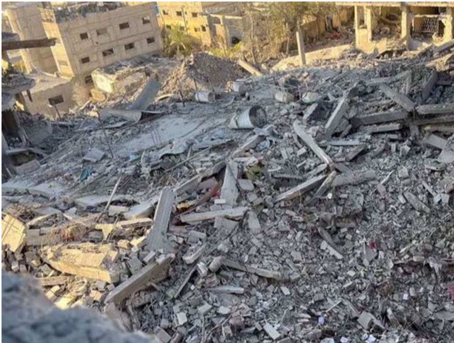
A multistory residential building lies in ruins following an Israeli attack in Beit Lahiya in the
