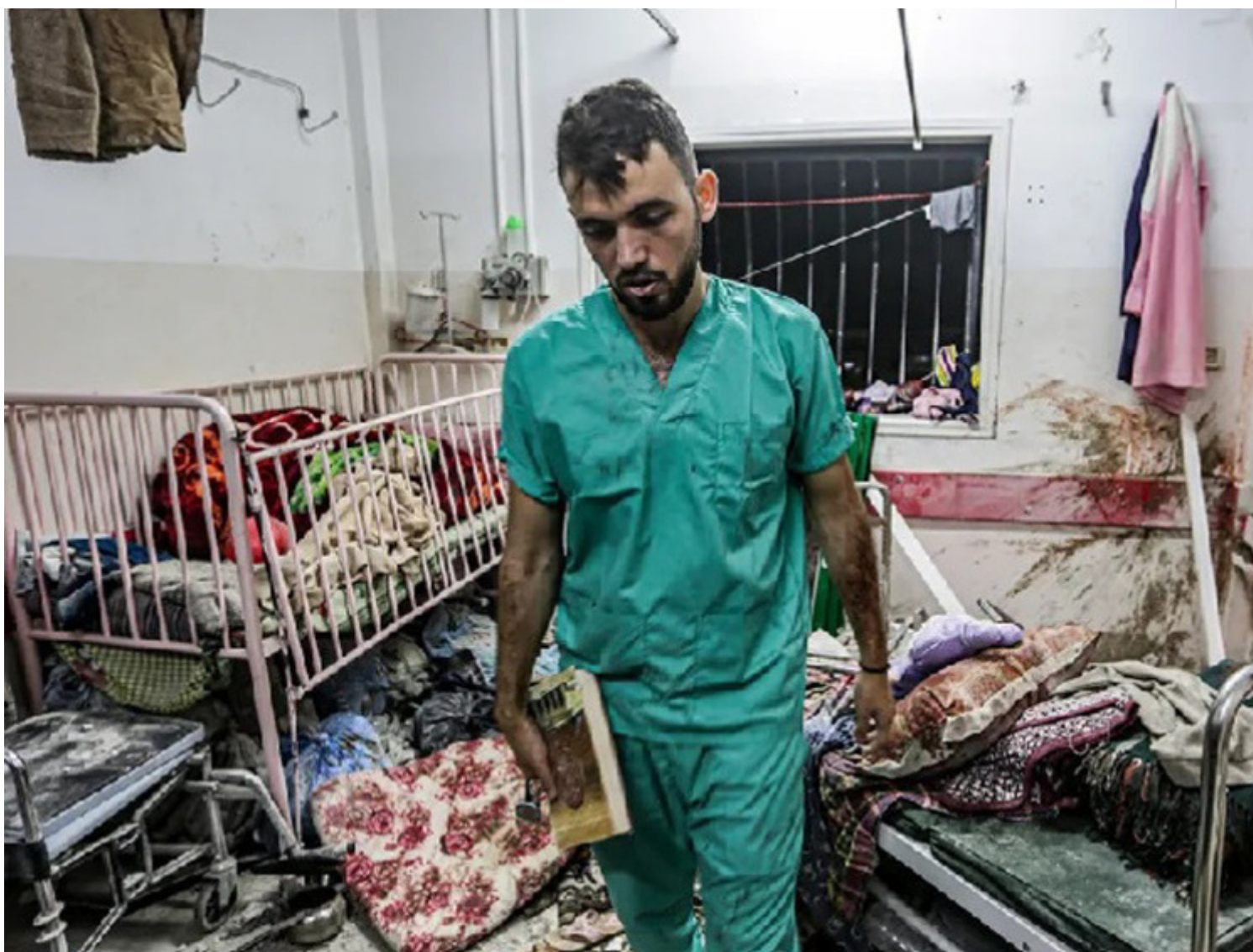
A man inspects the damage in a room at Nasser Hospital in Khan Yunis in the southern Gaza
