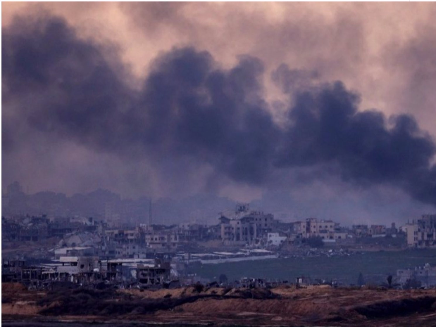
Smoke rises above destroyed buildings in the northern Gaza Strip during an Israeli army
