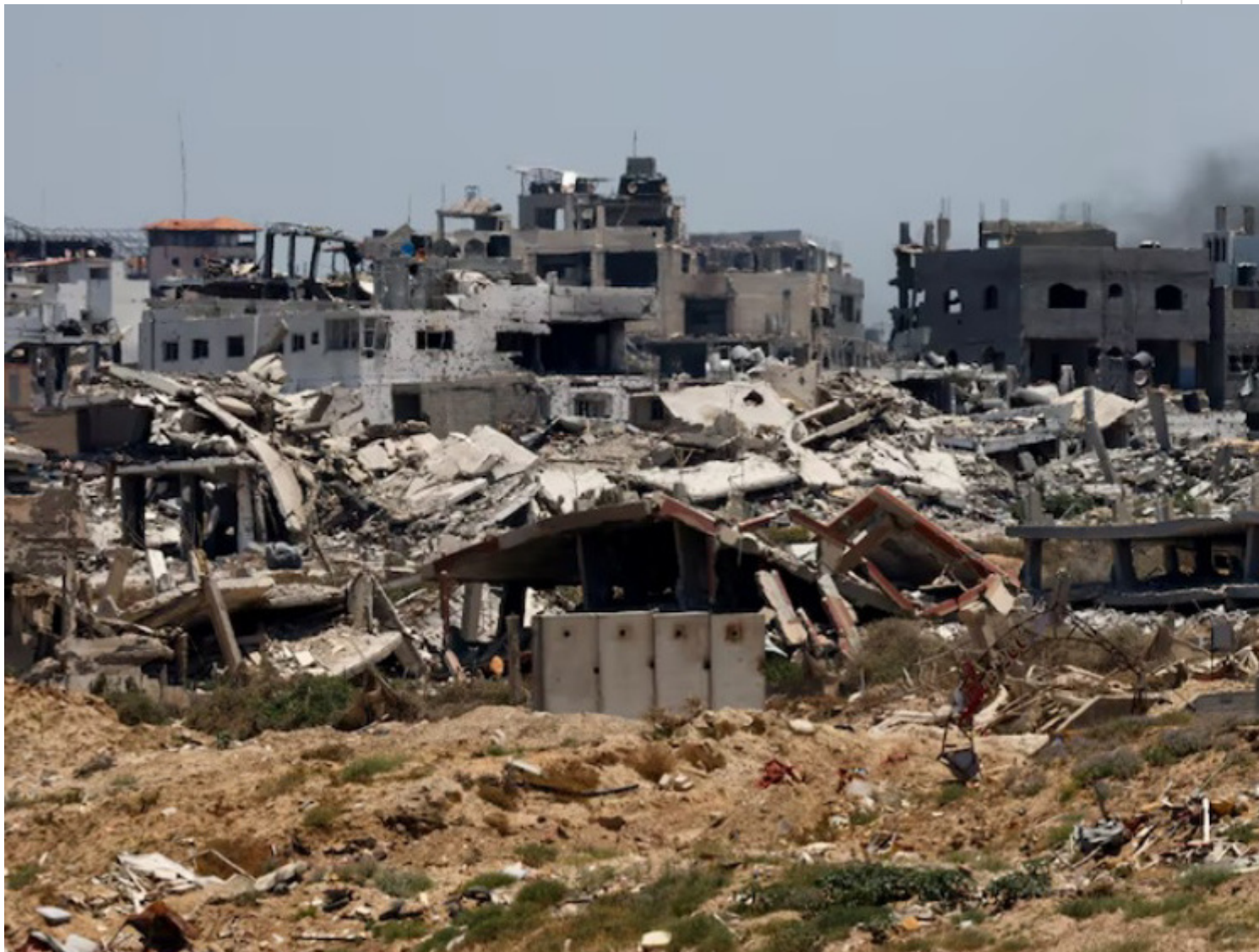
Destroyed buildings are pictured in Gaza, amid Israel's war on the Gaza Strip, on June 25, 2024.
